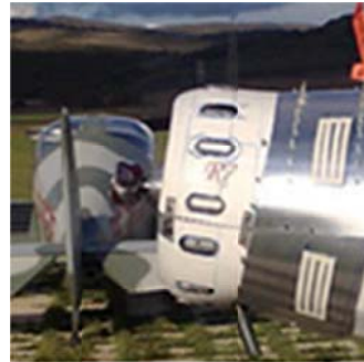
Vents (4off) being installed
